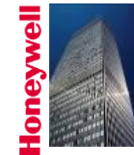
Environmental Control Systems
